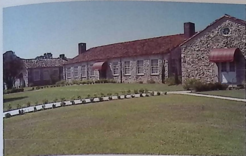
Fessenden Elementary School, Ocala
