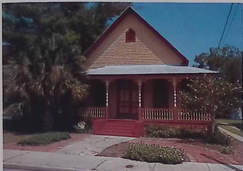
St. Michael's, Pensacola
