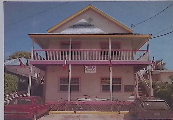
Caribbean House, Bahama Village, Key West
