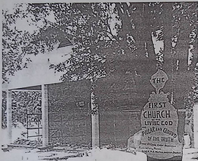
The New Church Temple Under Construction
