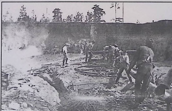
Workers moving hydraulic mining pipe in the mine pit. Note condition of pit bottom. Photo from the author's collection.
