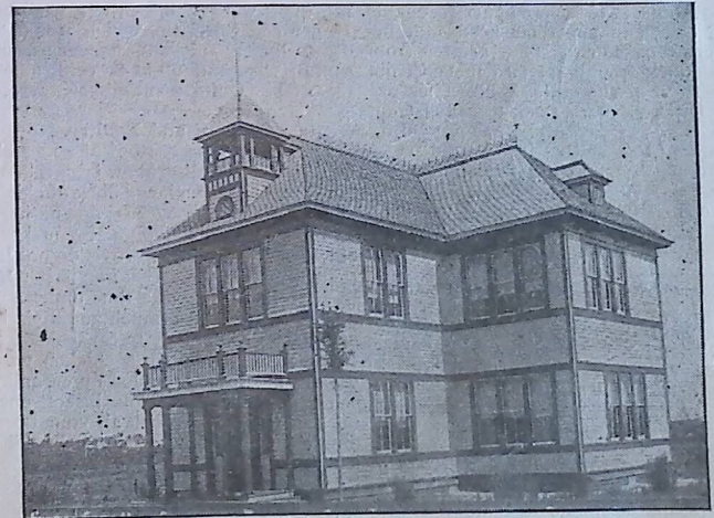
The High School Building, Floral City.
