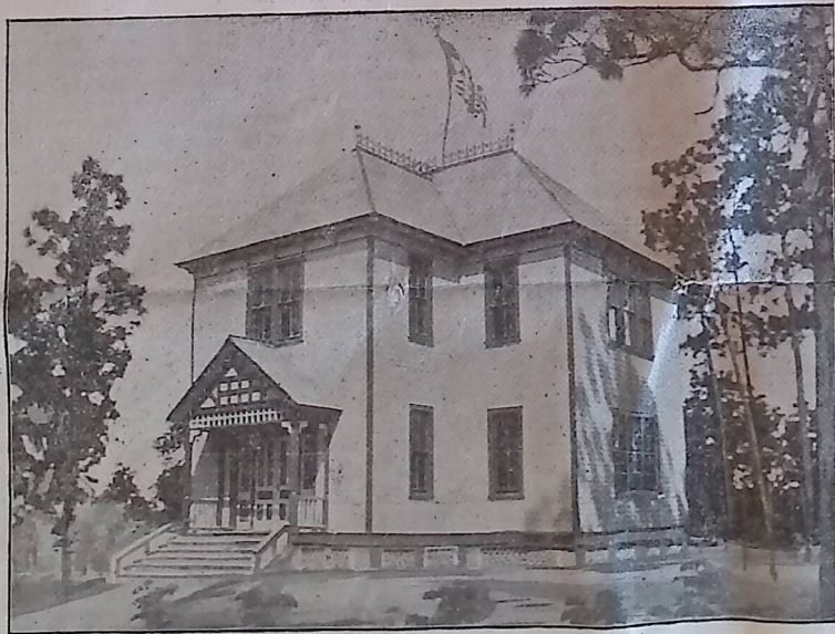
GRADE SCHOOL BUILDING.
